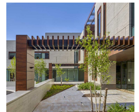
Patients arrive through a hotel-like drop-off area and garden. The garden surrounds the building and toggles between formality and simplicity, eventually giving way to clinical spaces.
